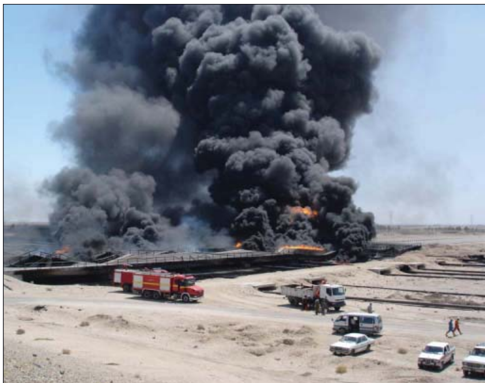
Iraqi Oil Pipeline Co. repair crews assess a damaged line. OPC is responsible for the maintenance and operation of Iraq's domestic pipelines (Fig. 1).
